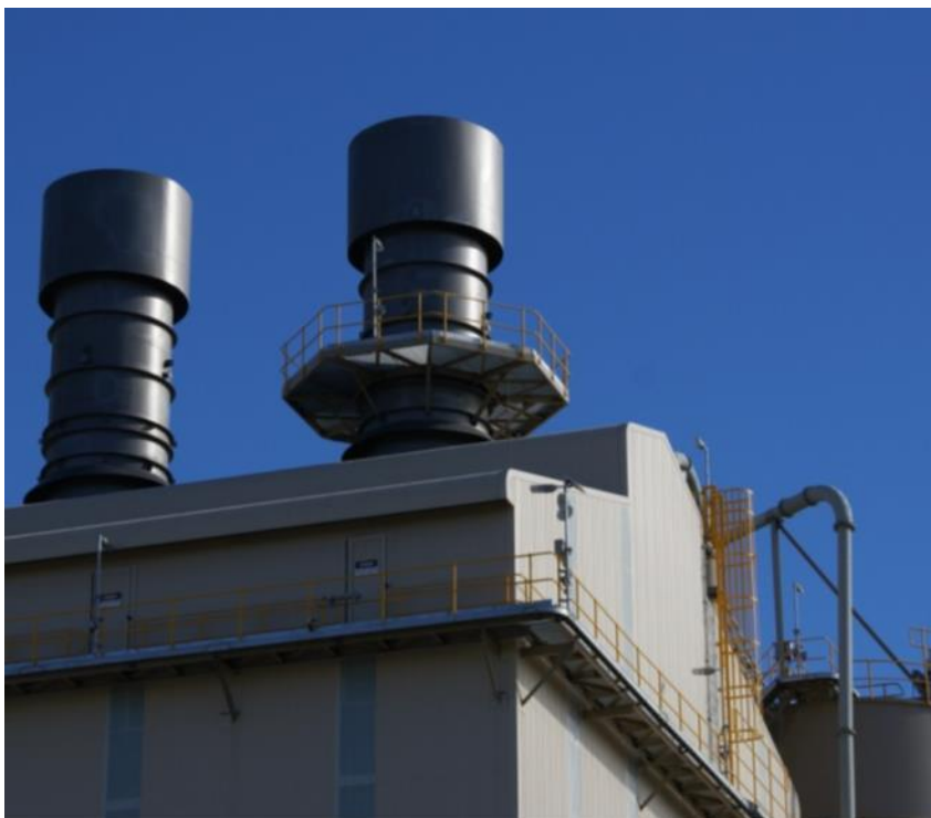
Figure 9: Sampling platform compliant with AS4323.1 constructed on the 3rd Furnace Baghouse stack
