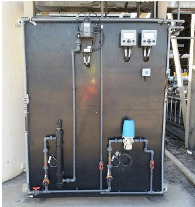
Figure 13: Continuous monitoring station for quality monitoring of transferred wastewater (input/output reference point W1)
